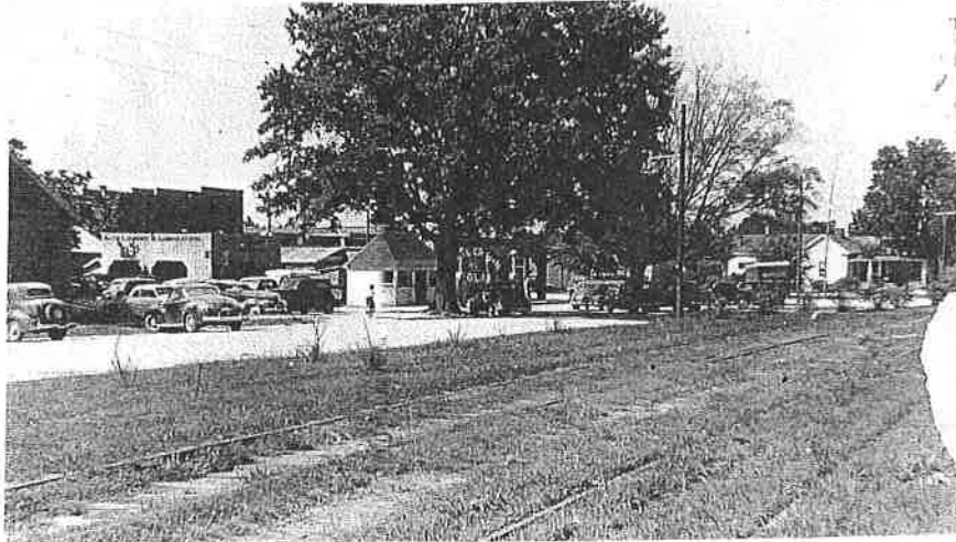
Views of the town: Top, The old R.L. Corbett Garage (also used as stables), Center, view of left side of HW #124, inside Macclesfield, where Penders Kwik Mart is today, Bottom, view from railroad tracks down the street where Southern Bank stands today.
