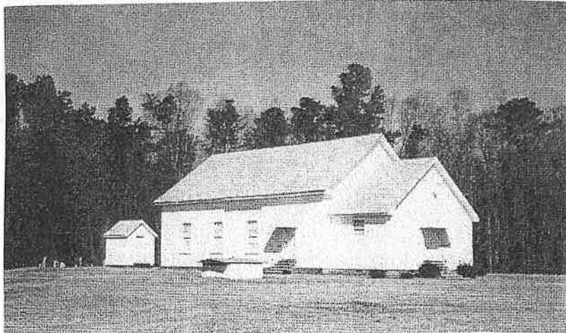
Maccripine Freewill Baptist Church
