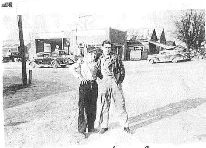
Old Service Stations in Town: Top and Center, the old service station located where the Kwik Mart is located today. Bottom, old service station in back of Eugene Eason and Graham Phillips.
